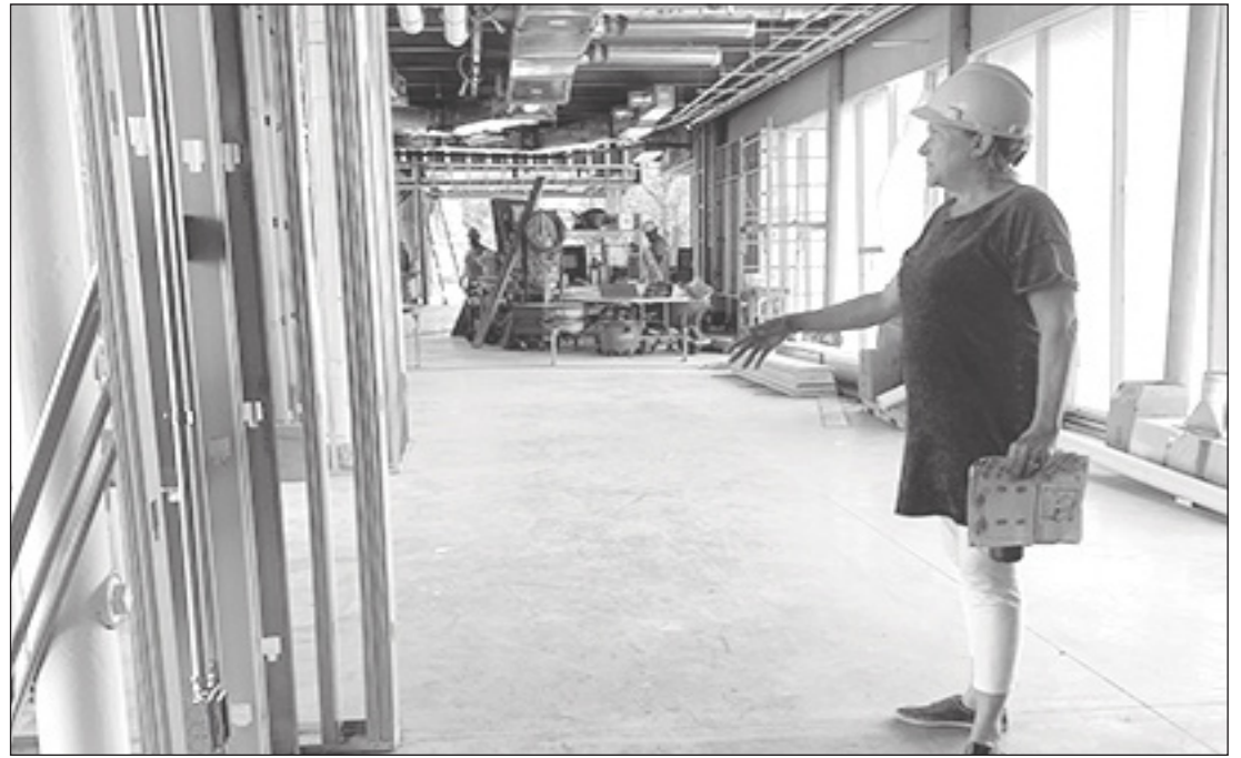
PHOTO BY CAITLYN NELSON | The Doane Owl Library director Joy Stevenson gives a tour of new library and shows progress made to new building.
